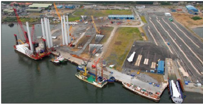
Offshore wind development can create jobs, as it did at this U.K.-based port.
